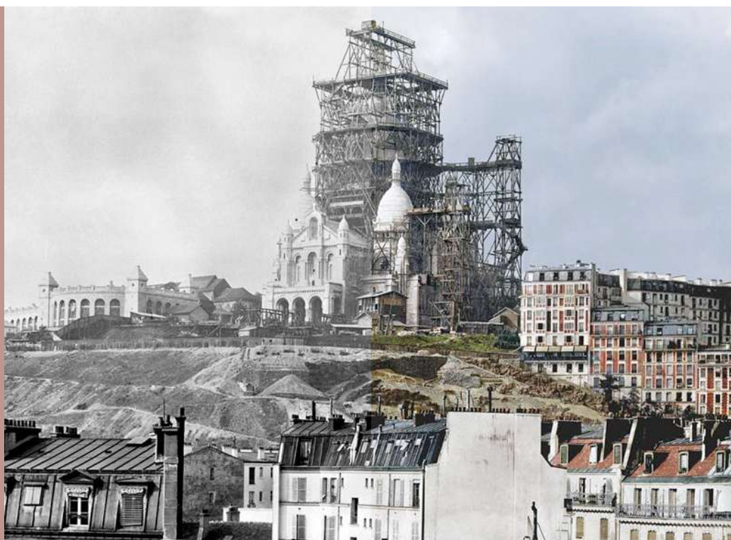
Construction of the Basilica dedicated to the Sacred Heart in Paris (Montmartre), photo of 1890
